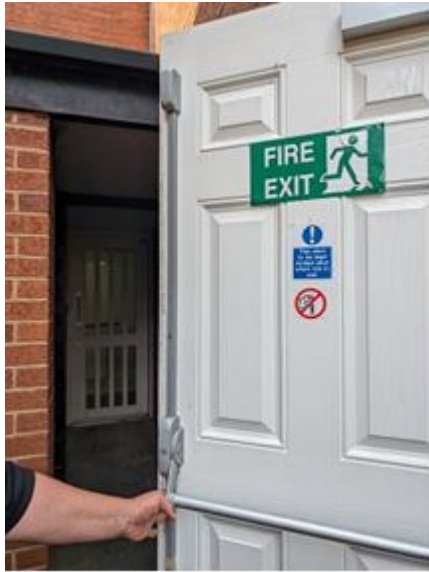
Fire door exit with push handrail.
