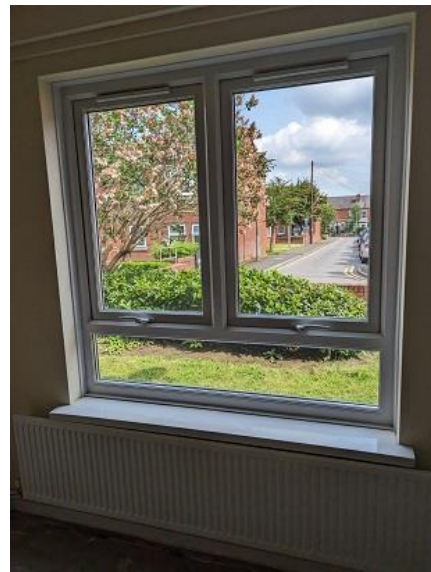
Accessible window openings
